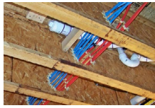
PEX WATER SYSTEM The Schumacher Way
